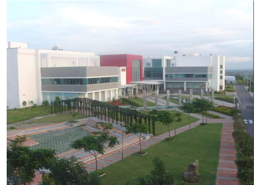
The Materials and Biosciences buildings at DKC
